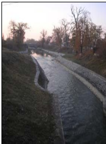
Figure 3: The Bega River/Canal downstream the Coștei dam house.
