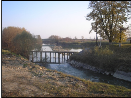
Figure 1: Coștei hydrotechnical diversion system area.
