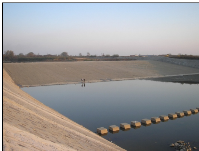
Figure 5: Coștei Dam on Timiș River; no water was left to flow over the dam.
